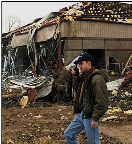
Michael Goodman, KD5FAQ, in front of the brand new Beebe Junior High School building destroyed in the January 21 tornado, assists with health-and-welfare traffic.
