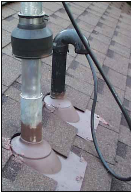
Figure 3—With the flexible rubber drain connector raised, portions of the mast and tower sleeve are visible. A piece of two-inch aluminum no-caulk vent-stack roof flashing with a neoprene seal placed over the tower sleeve prevents water from running down the outside of the tower sleeve and into the attic. Nearby, the coaxial cable feed line passes through an added vent pipe and elbow on its way from the attic to the antenna.
