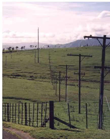
What appear to be telephone poles are actually supports for the feed line to the rhombic antenna. Title photo: The station building at Quartz Hill.
