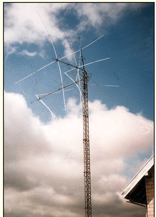
This used to be a 4-element, 40-meter quad antenna. It was the pride and joy of Krzysztof Sobon, SP7GIQ, in Lask, Poland until a storm brought winds exceeding 110 miles per hour.
