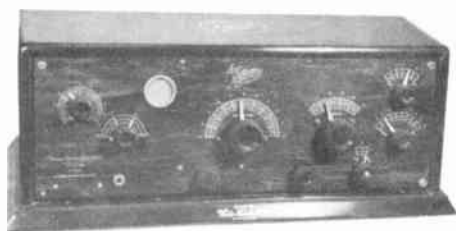
ZN-1TH 3R LONG DISTANCE RECEIVER CHICAGO RADIO LABS. NL 1923 S.P. $160.00
